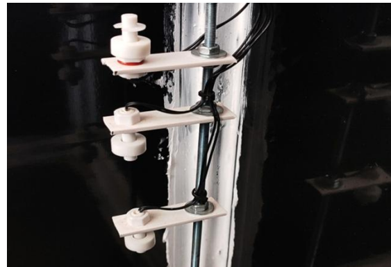
Fig. 4: Float switches inside the water tank.
